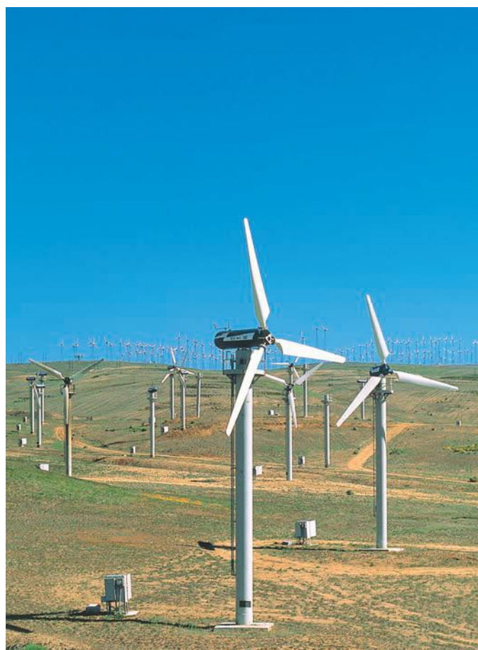
Figure 21.31 Wind generators in the USA. On otherwise unproductive land or offshore, these generators make an increasing contribution to the electricity supply.
